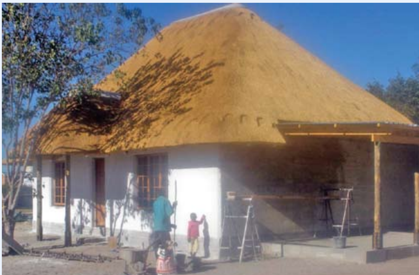
Figure 7 - Partially completed house.
