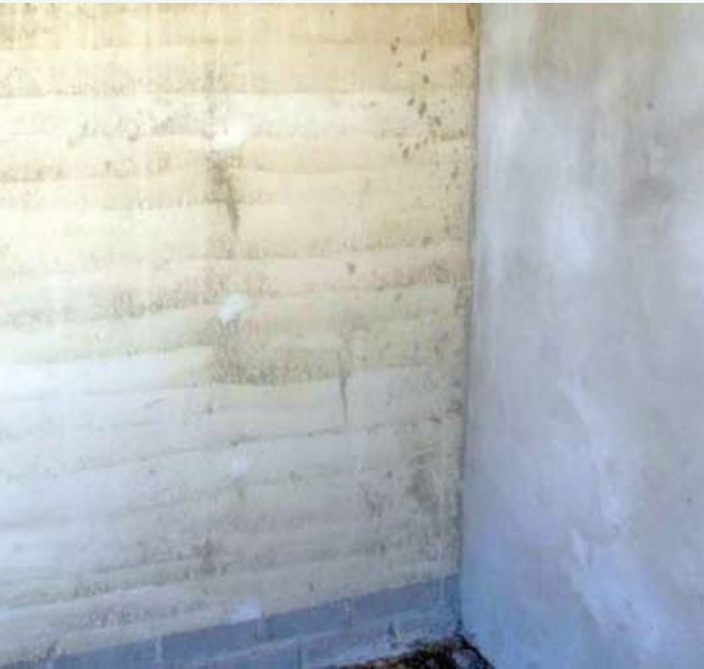
Figure 5 - Partially plastered rammed earth wall.
